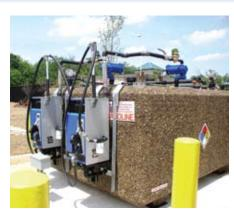
Capturing the best of large fleet dispenser performance in a compact design, the Reliance® S1 fuel dispenser is ideal for Aboveground Storage Tank (AST) applications. Its small cabinet attaches easily to an AST shelf, yet it features the same capabilities as standard full-length cabinet fleet dispensers.
